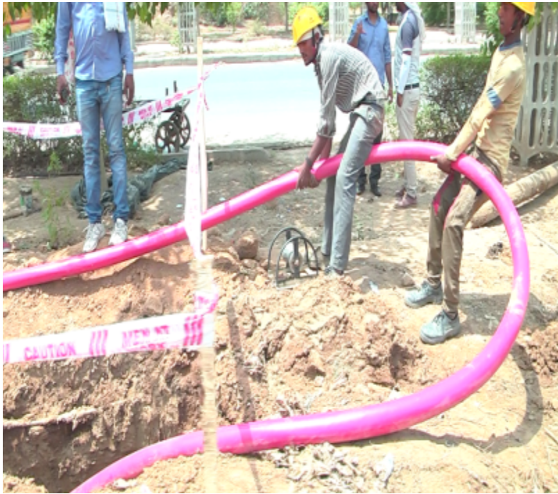
Helpers pulling cable from the drum
