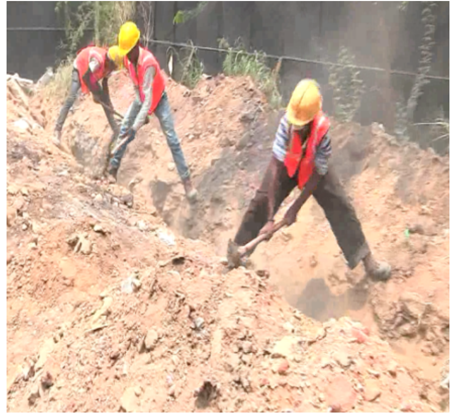
Filling the trench with hard soil
