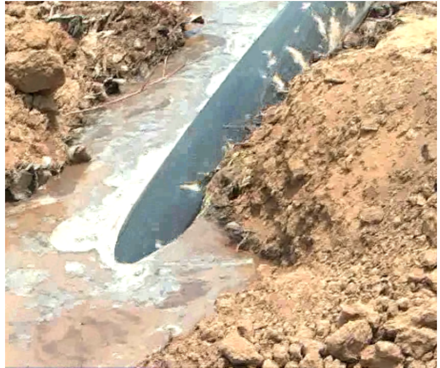
Insertion of HDPE pipe through bore
