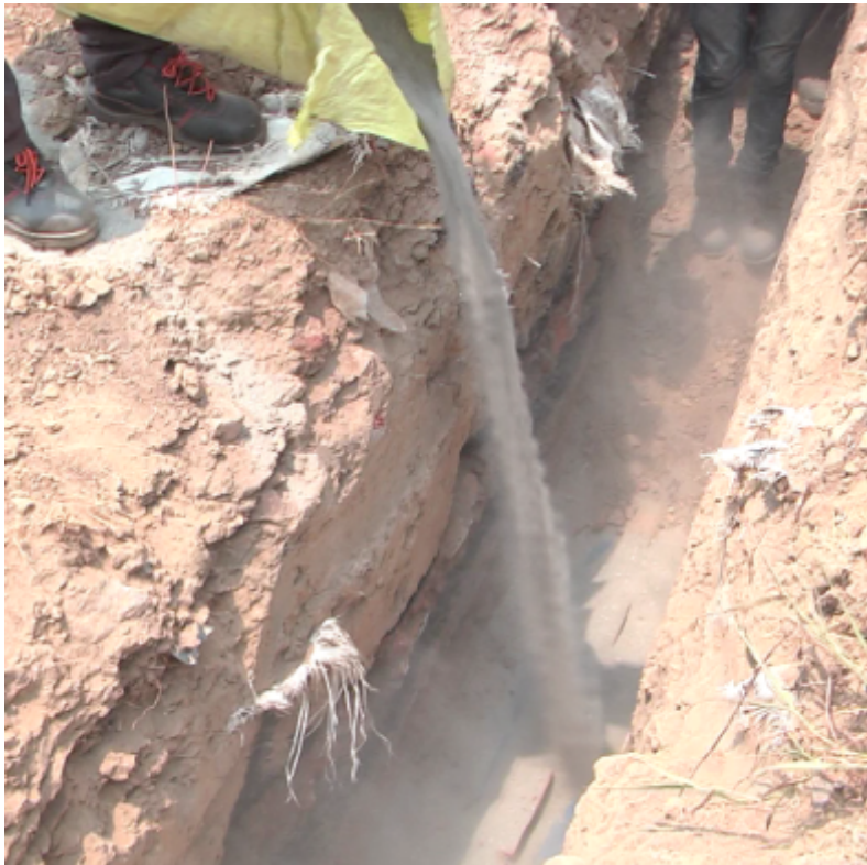
The trench being filled with soil
