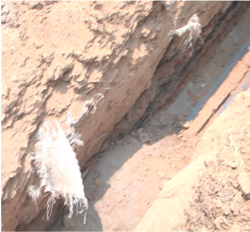
Excavated trench for double circuit
