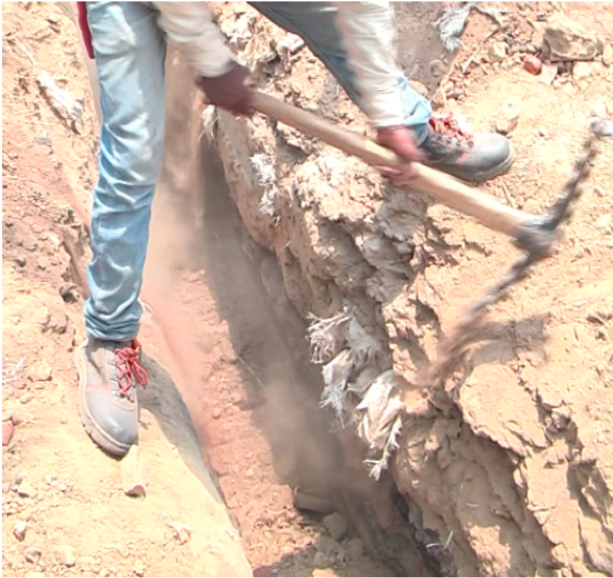
Filling the trench with soft soil first
