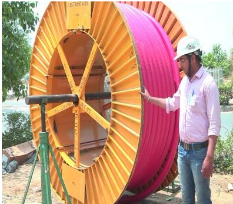
Cable attached to the drum jack
