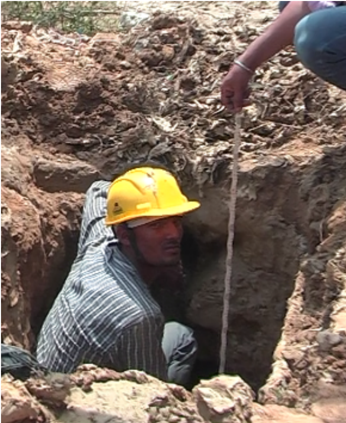
Test pit of cable trench
