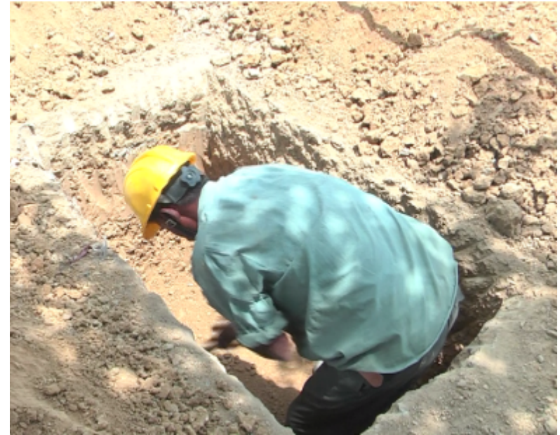
Digging a pit for laying trenchless cable
