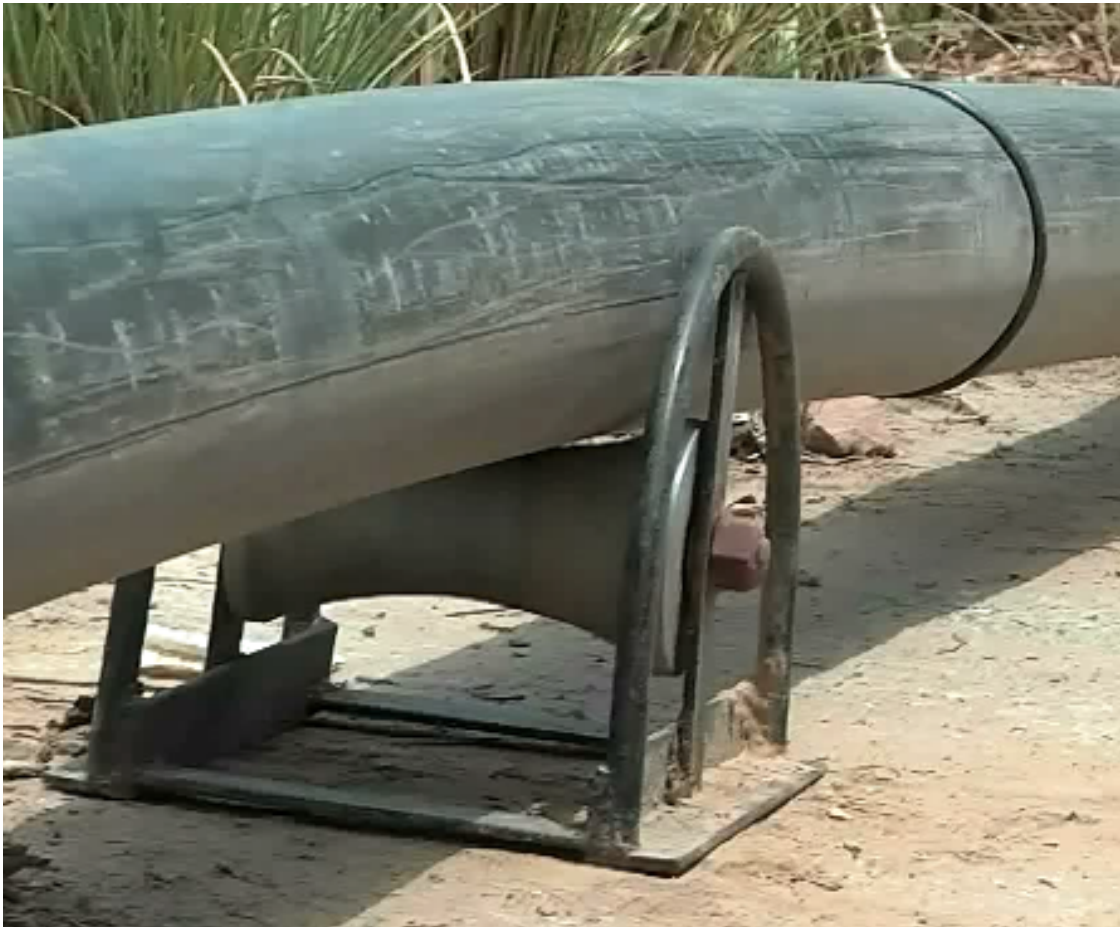
Roller stools for smooth movement of the pipe
