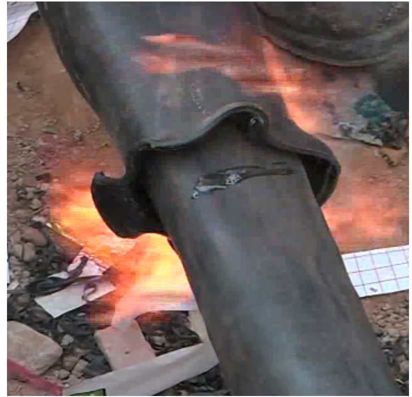
Heat treatment process of straight through joint
