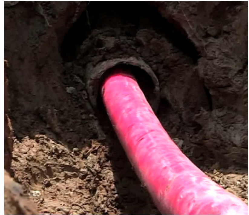
Cable going inside the pipe
