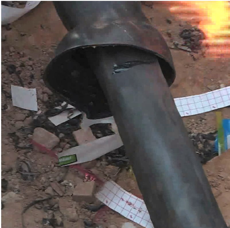
Heat treatment process of straight through joint
